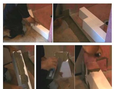
Use your corner-installation techniques to install these at each end of the curb. Finally, measure and cut a proper sized piece of membrane to cover the curb. Ensure that there is a minimum of a 2" overlap onto the pan floor. Install like other membrane sections.
