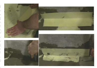
17. After completing all lower horizontal joint strips, proceed to installing vertical joint strips using the exact same techniques. If you are not taking your tiling all the way up to the ceiling, be sure to mark where your tiling will end and measure the correct length for each piece. Repeat for any vertical corner surfaces. Note: If you run short on band, you can create your own out of any excess membrane.
