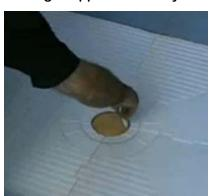
3. Drill Pilot Hole on the inner circle you have hand drawn Use the jigsaw to cut hole in subfloor using the innermost circle as a guide (~4" diam.). There should be enough clearance for the tail-piece of the drain flange, but the base of the flange is preferably supported by the subfloor. Be sure to (test) dry fit drain flange and pan pieces.
